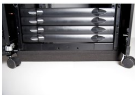
Expanded foam seals beneath a rack.
